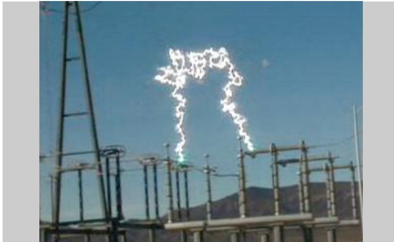
A 500 kilovolt circuit breaker reveals the concentration of destructive energy possible at a double layer.
